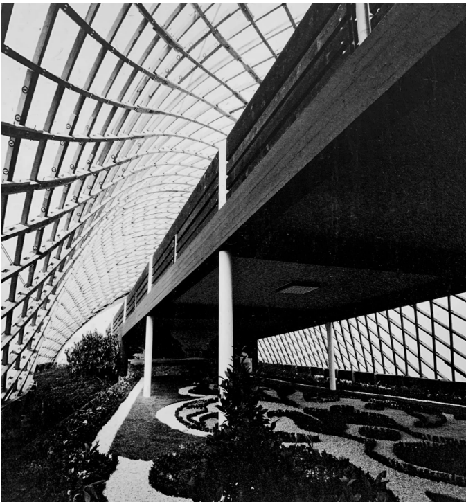
Figure 3: Historical images of Multihalle with one of the entry ramps and the view from above, 1975.
