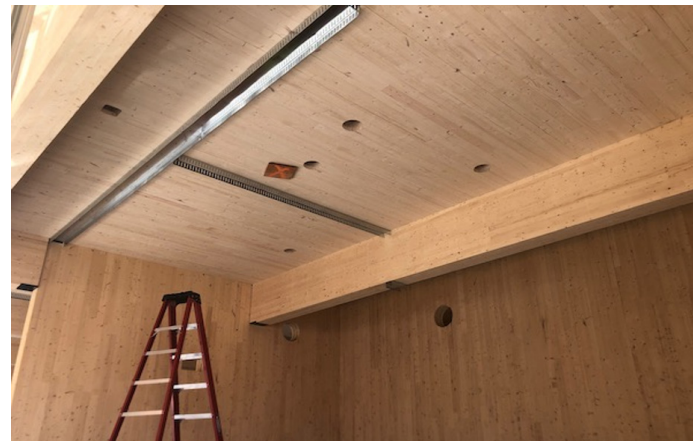
Figure 1: CLT Ceiling panel with pre-drilled penetrations
